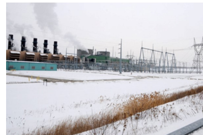
Midland Cogeneration Plant Source: Midland Cogeneration Venture
