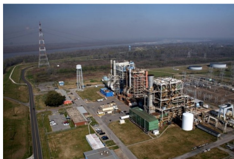
Little Gypsy power plant Source: Entergy
